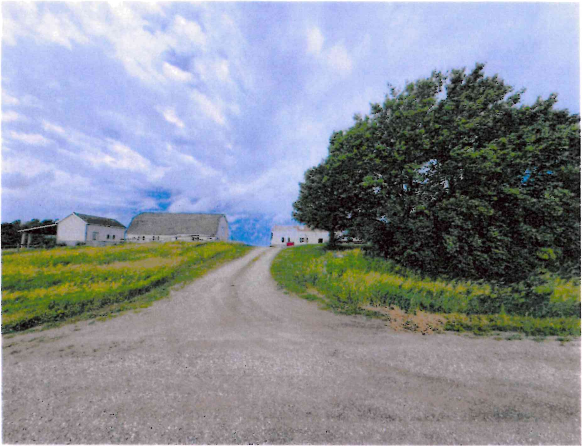
Figure 4 Building Site at 11332 Killdeer Avenue
