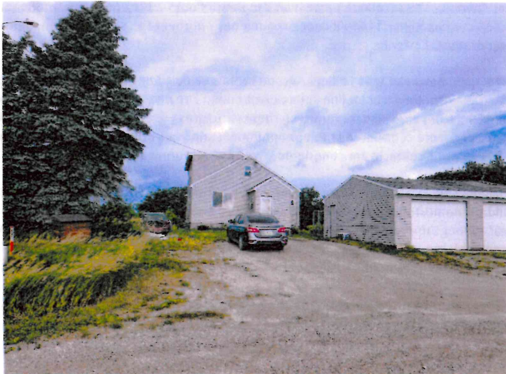
Figure 1 Building site at 11446 Killdeer Ave
