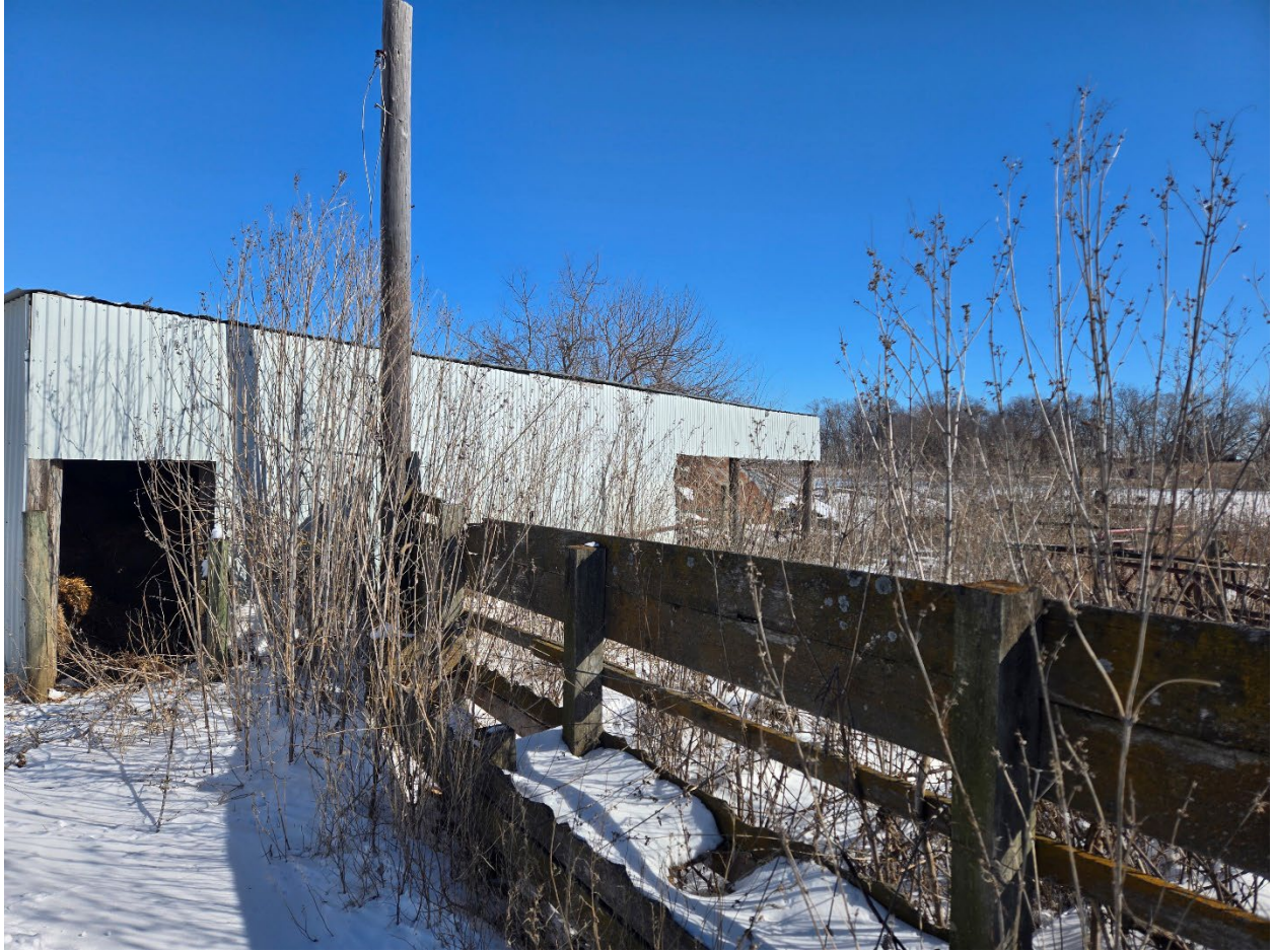
Figure 3 Northeast Machine Shed
