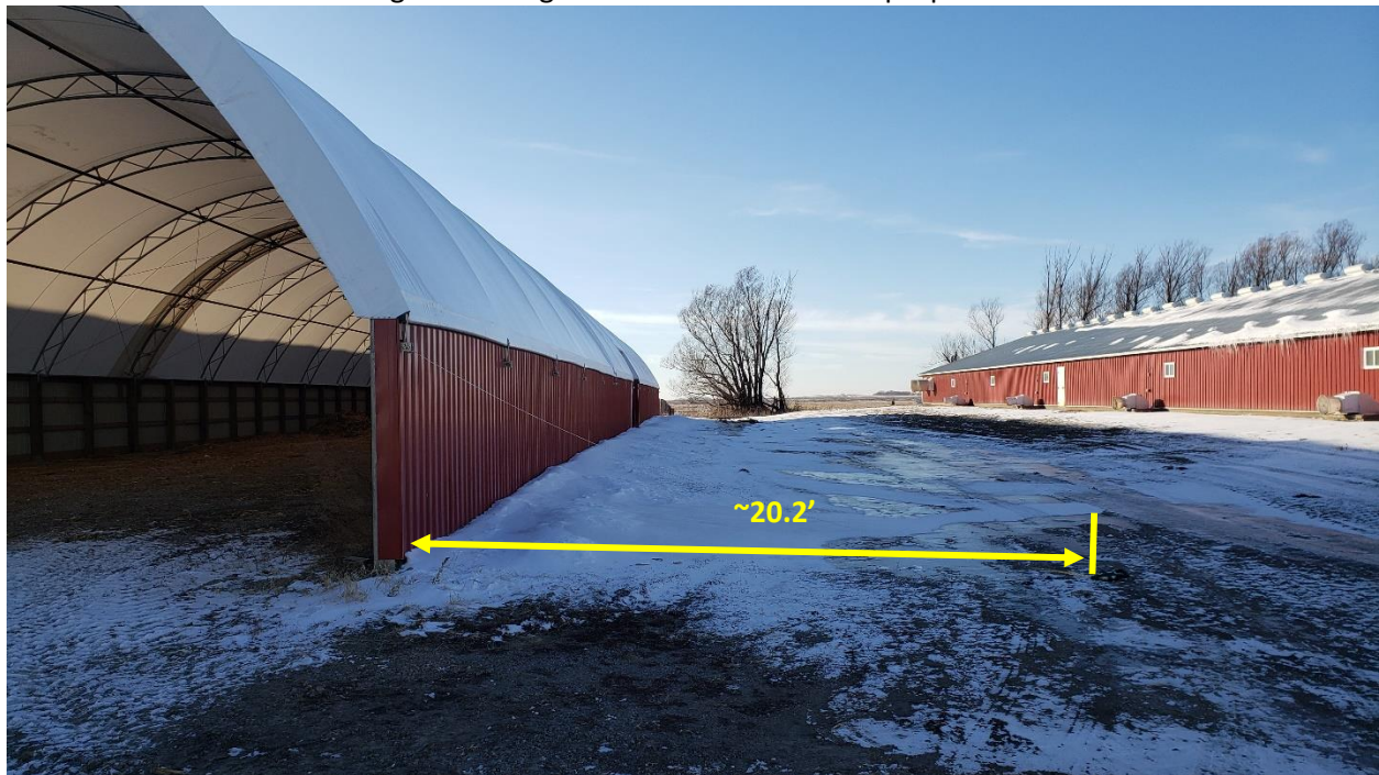
Figure 10 Looking west along the north side lot line of proposed Lot 3
