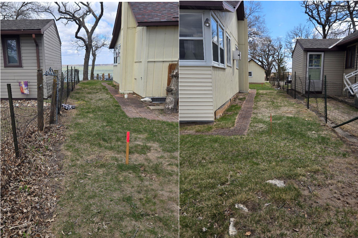
Figure 5 – Looking along the west side lot line from street and lake at proposed location of dwelling 4' from the west side lot line
