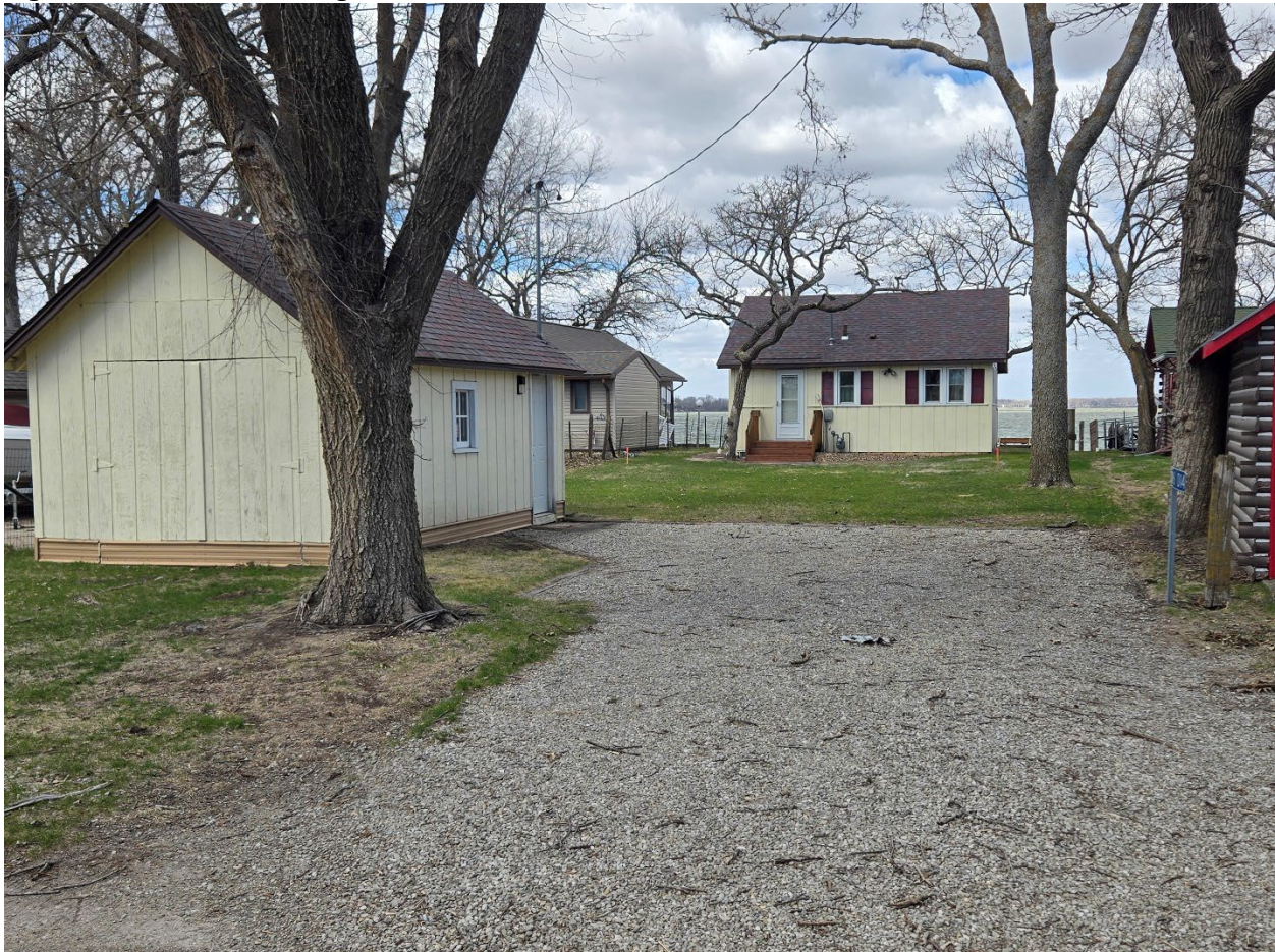
Figure 1 – View of existing cabin and shed on the lot
