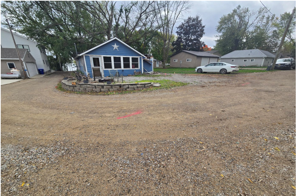
Figure 1 Existing cabin from Basswood Ave
