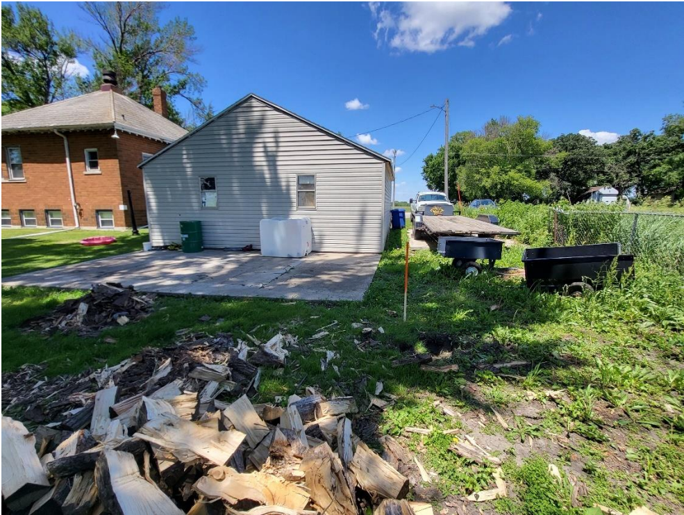
Figure 4 – looking south at proposed west side of garage footprint
