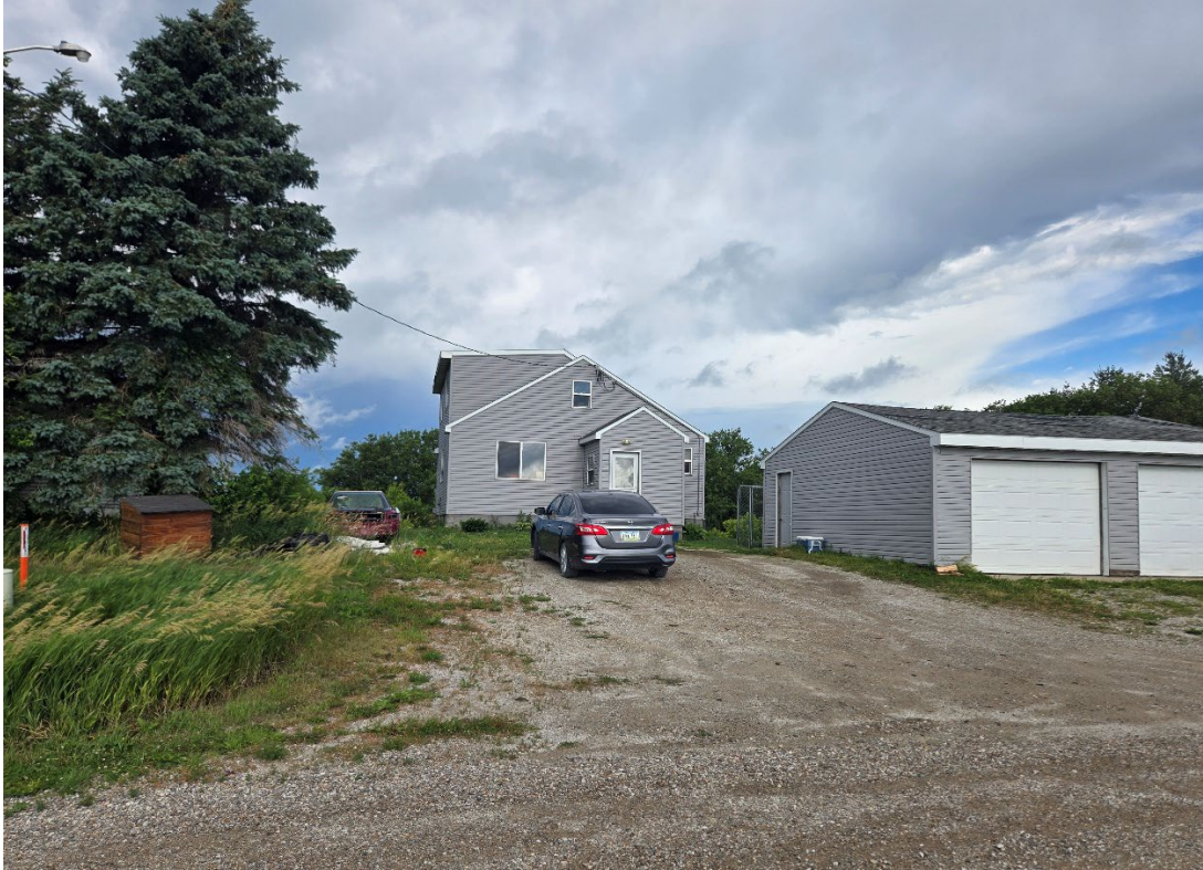
Figure 1 Building site at 11446 Killdeer Ave
