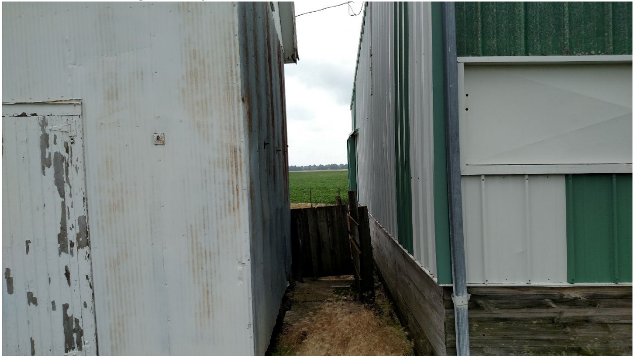
Figure 6 Looking at the separation distance between the two easternmost sheds
