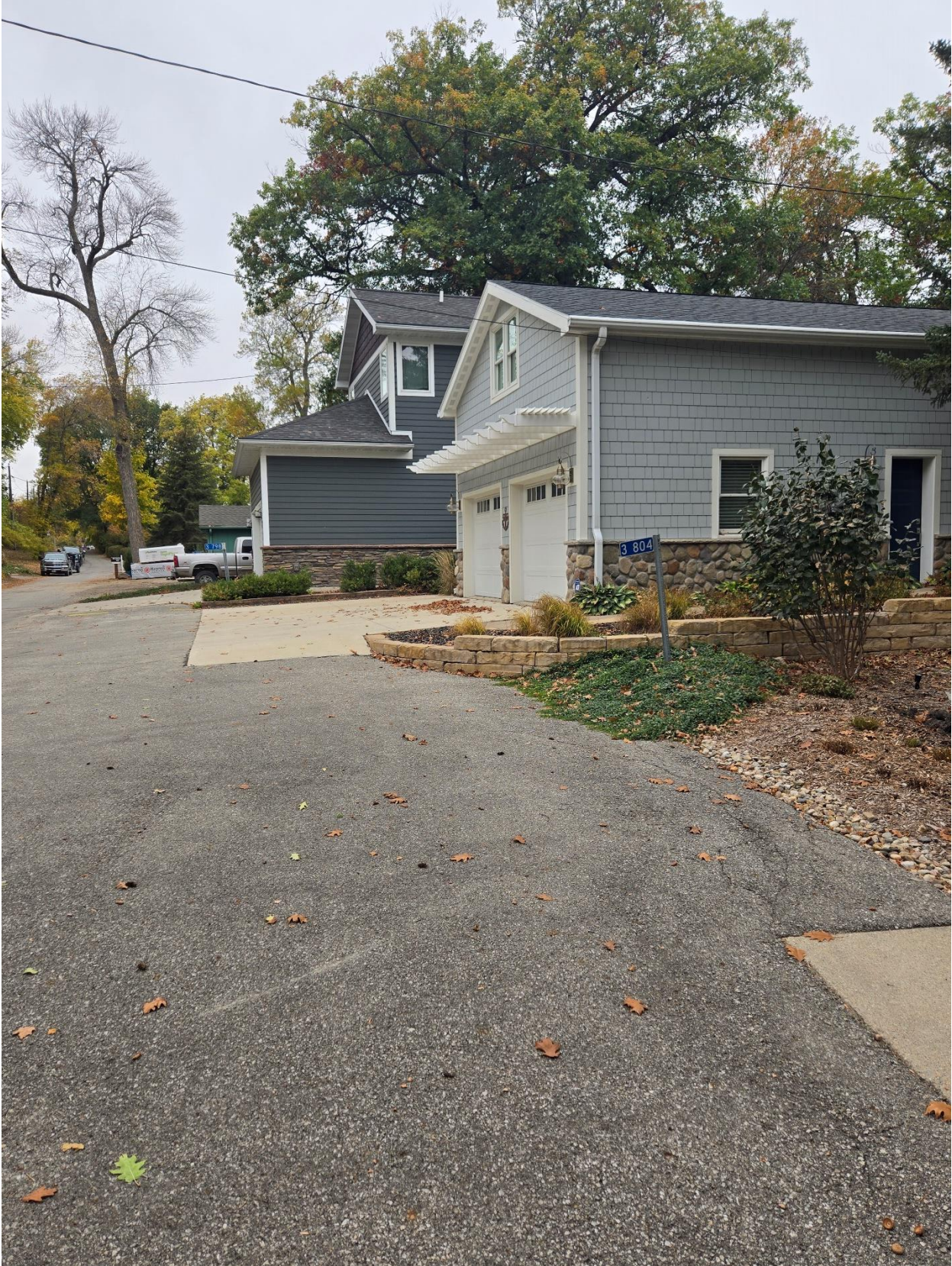
Figure 4 – looking west along the front building line of the garage
