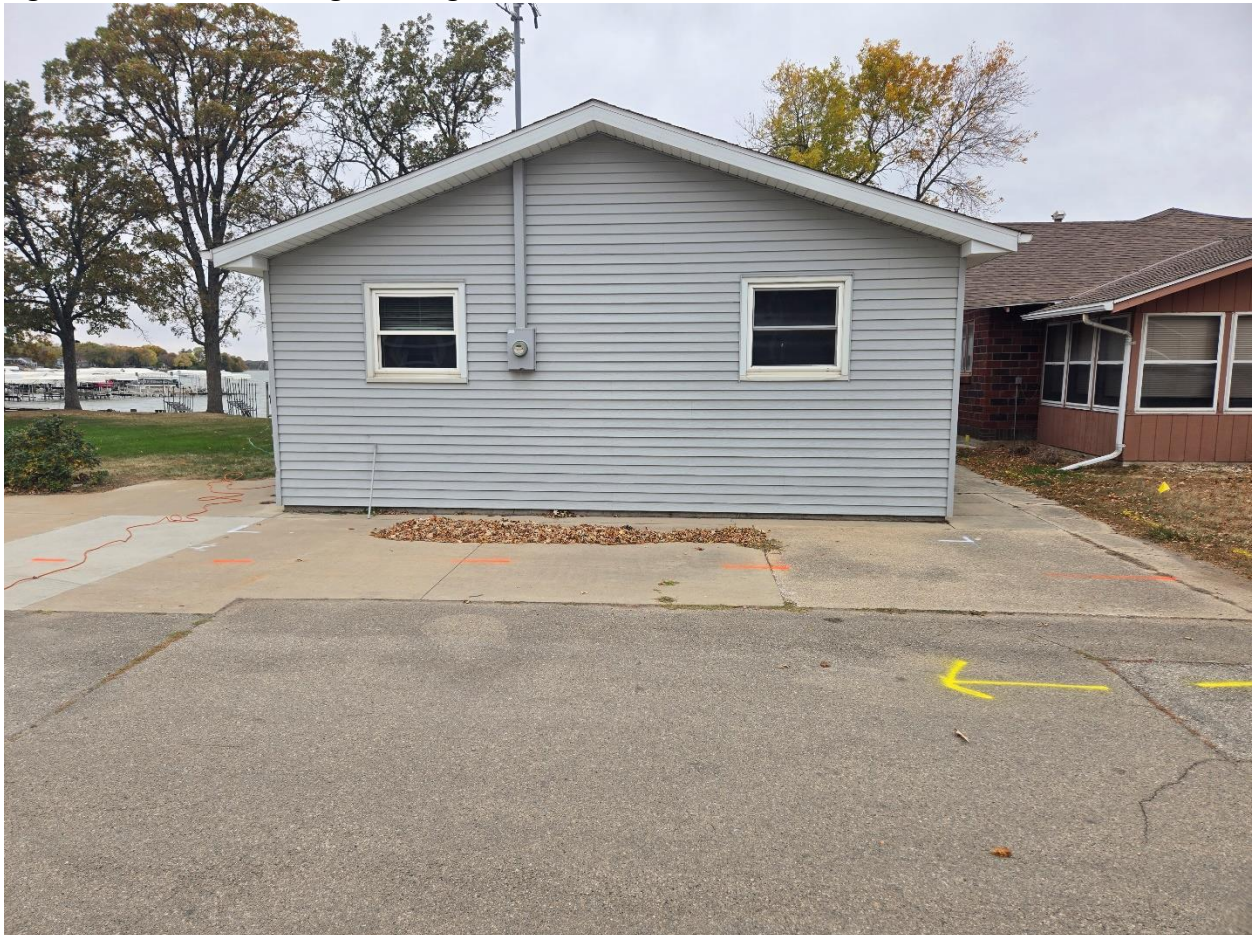
Figure 1 – View of existing dwelling from Lambert Drive
