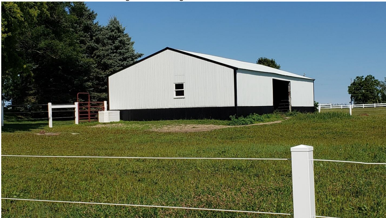
Figure 4 Looking at the existing east machine shed on Lot 1
