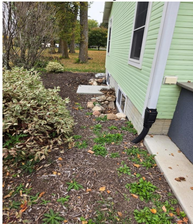
Figure 4 Rear of house looking east to west
