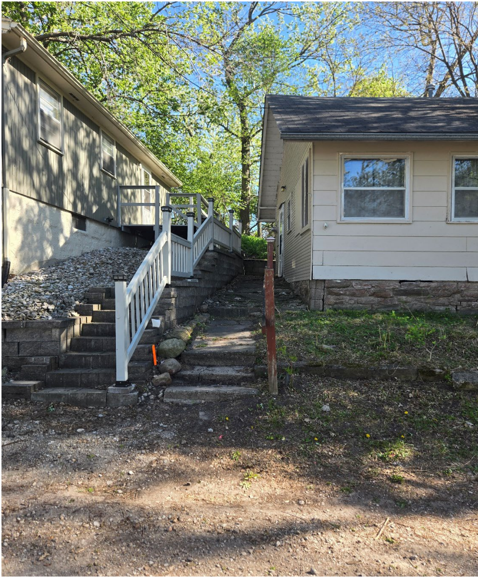
Figure 3 Looking along east lot line
