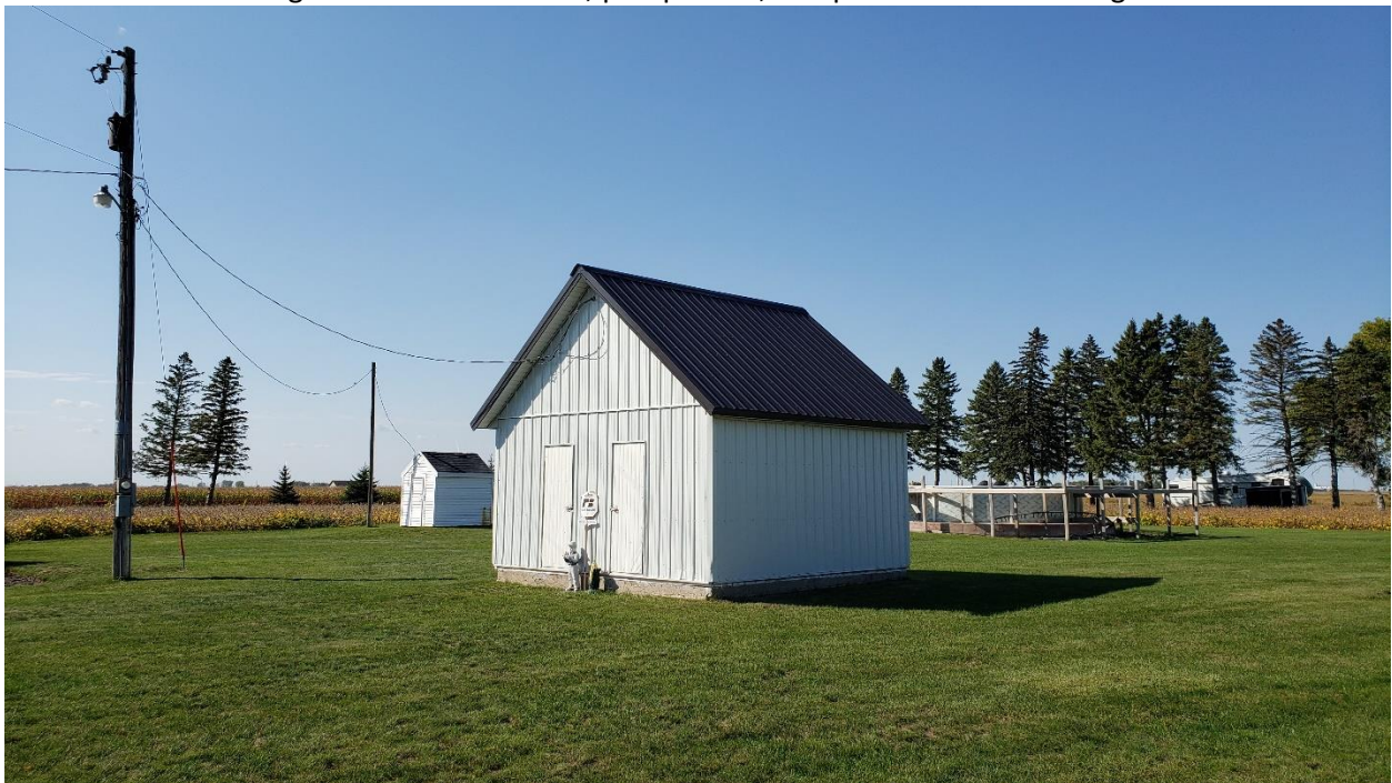
Figure 4 Looking at the southern shed, pumphouse, and pool with surrounding deck
