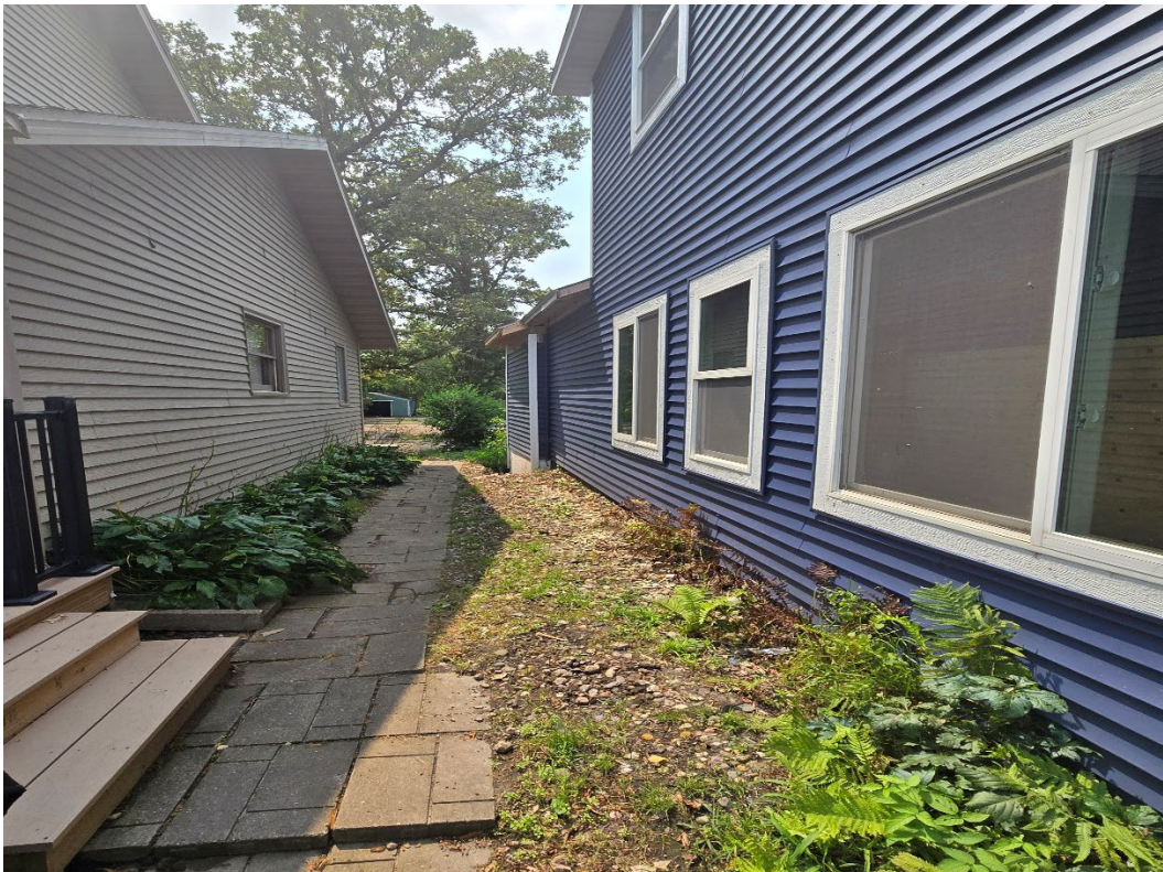
Figure 3 Looking south along east lot line
