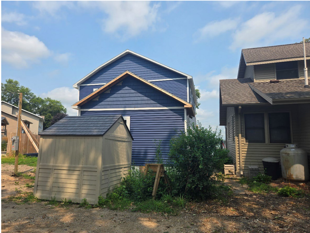
Figure 2 Distance between neighboring house to the east
