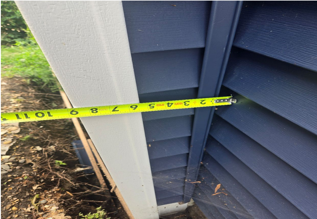
Figure 5 Measurement of well house addition
