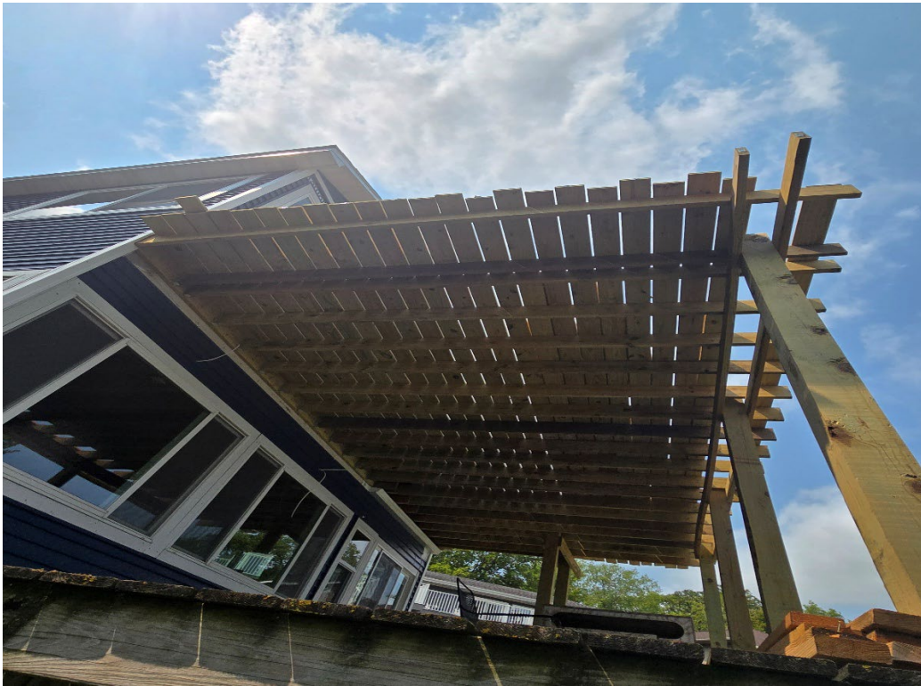
View of deck from ground level
