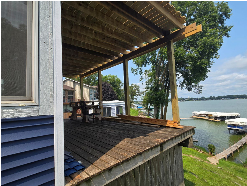
Figure 3 View of lower level deck to be screened in
