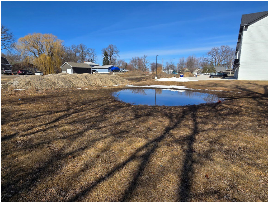
Figure 6 Drainage area behind Lake Ridge condos
