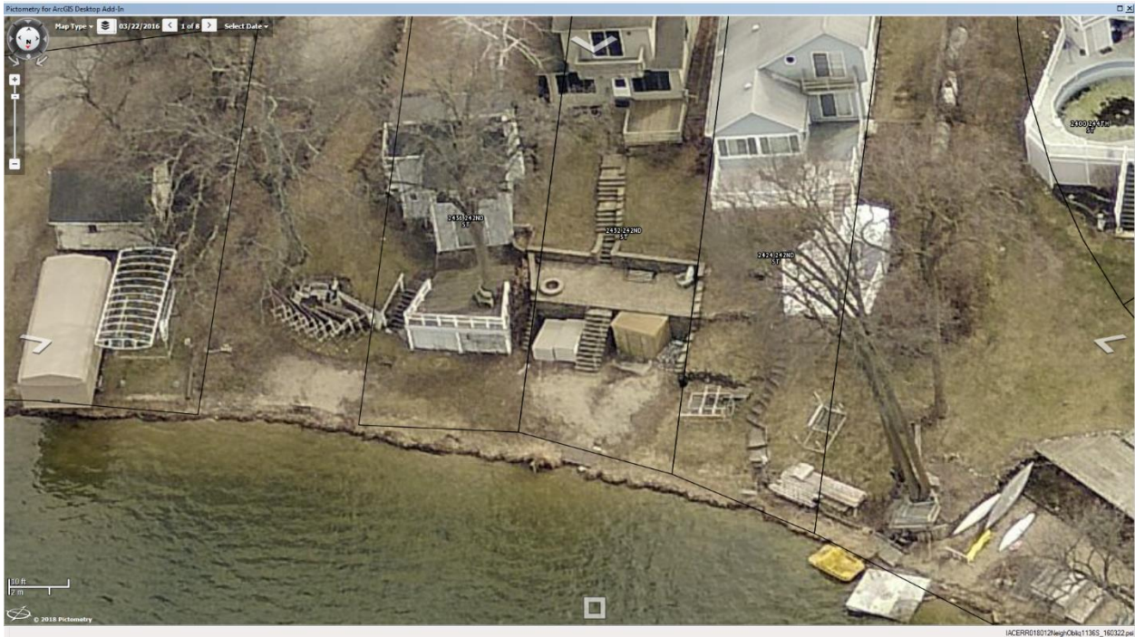
Figure 8 Aerial photo showing the lake side (rear) of the mentioned properties
