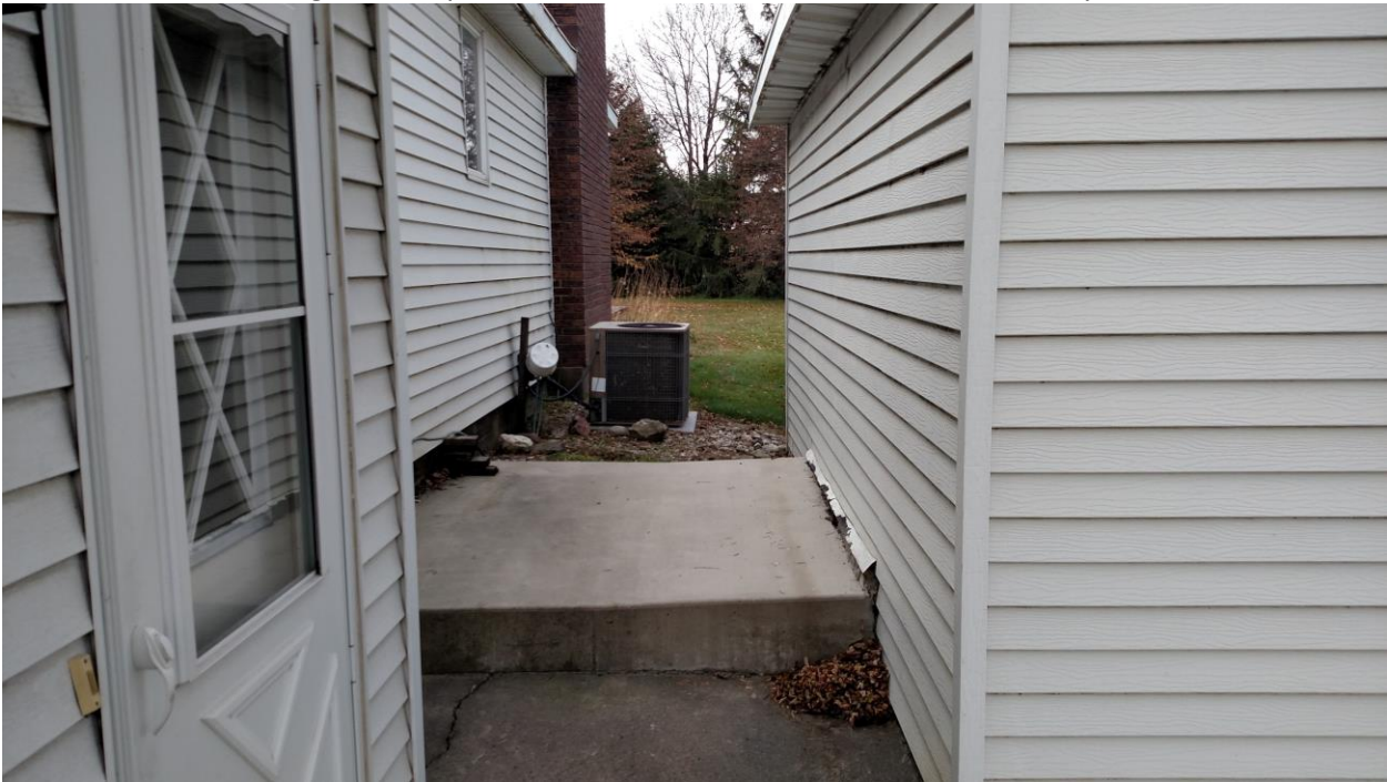
Figure 4 Looking at the separation distance between the house and nearby shed
