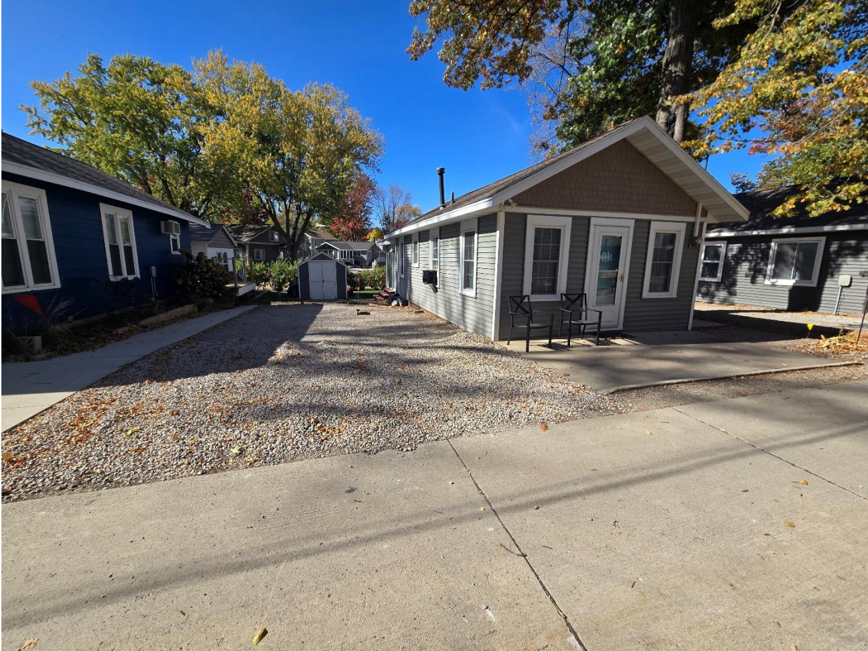
Figure 4 – Looking at distance between Ubben dwelling and dwelling to the South
