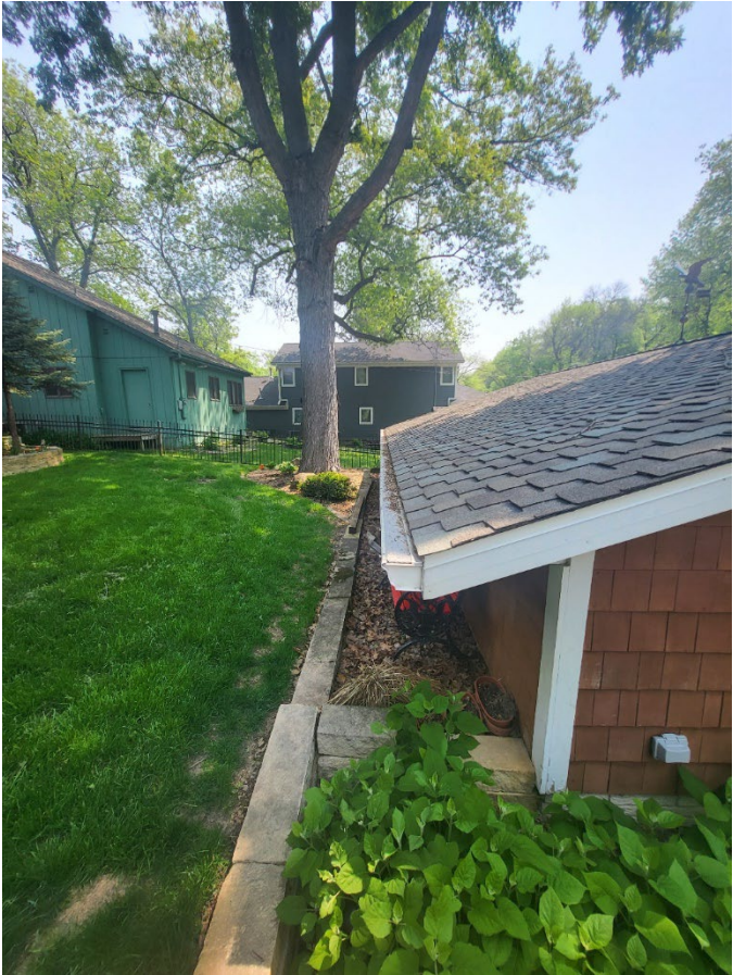
Figure 4 – rear of garage looking west to east
