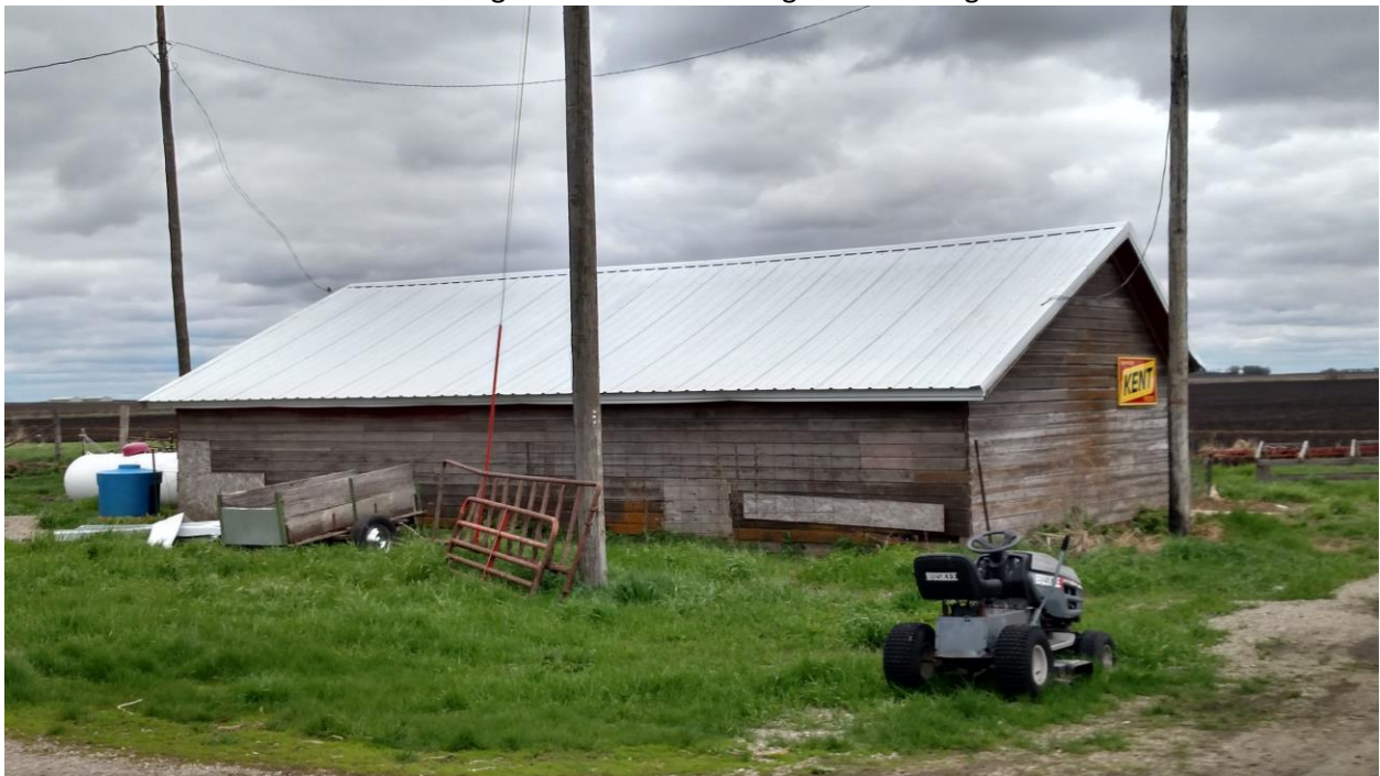
Figure 4 Looking at the central existing farm building
