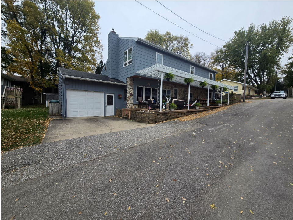
Figure 2 View of pergola looking southerly on Blacklocust Ave
