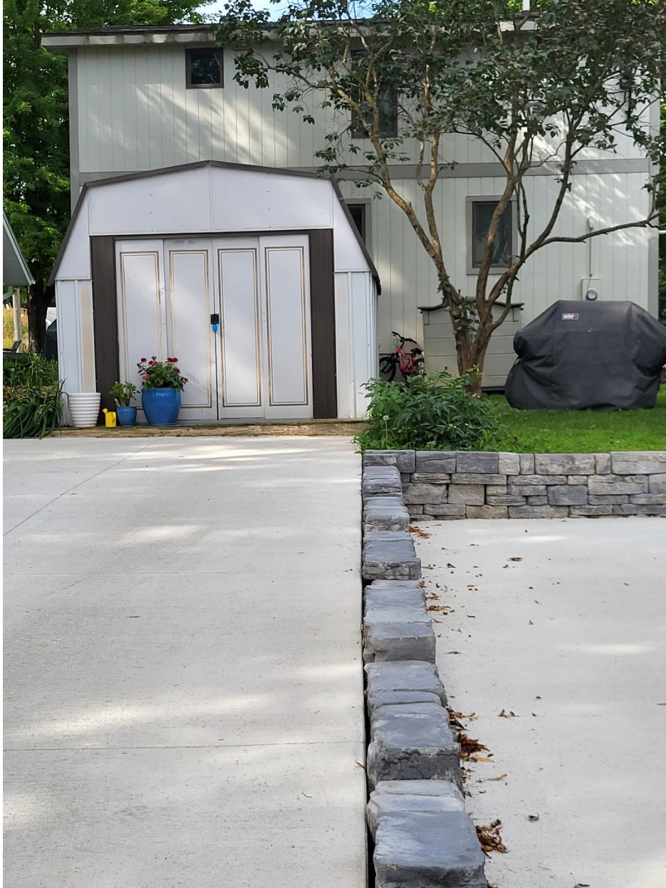
Figure 1 – Existing shed along the west side lot line
