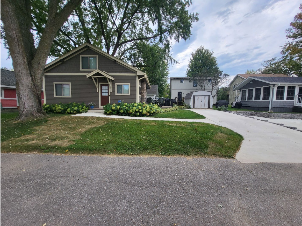
Figure 5 – View of property from 6 th Street
