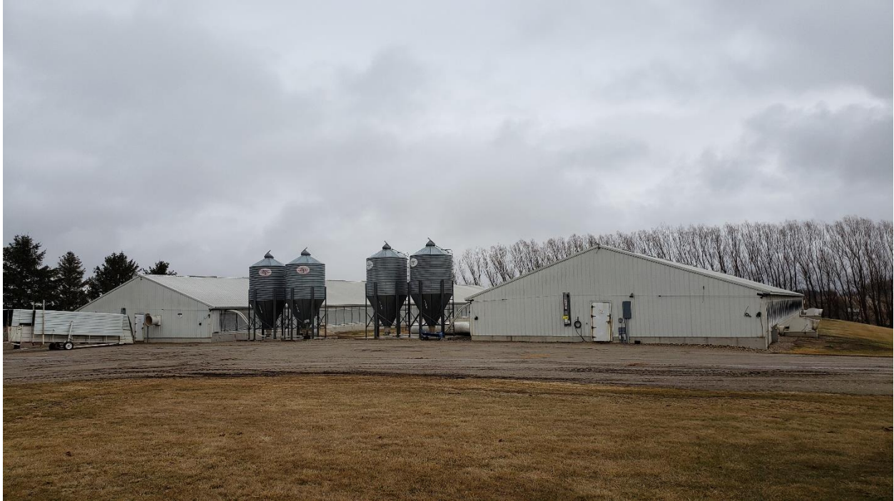
Figure 3 Looking at the two hog confinement buildings
