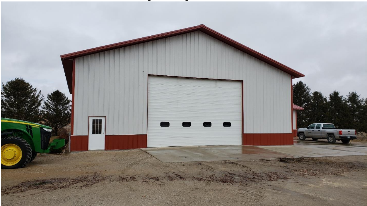
Figure 4 Looking at the large machine shed
