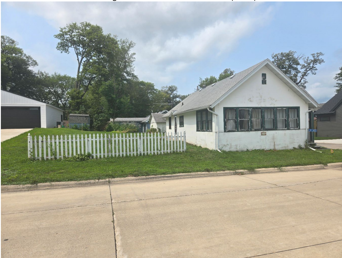
Figure 1 Existing house from Southshore drive (Front)
