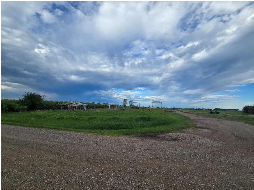
Figure 2 Hoists located on south side of driveway
