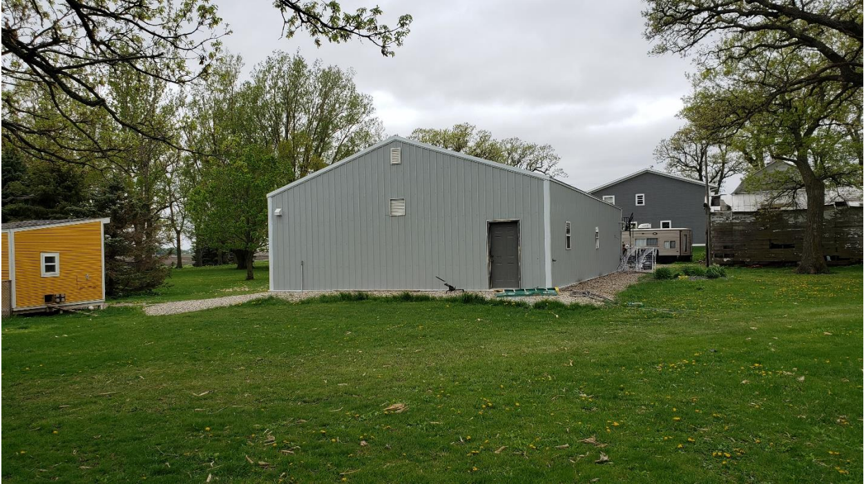
Figure 5 Looking at the existing machine shed
