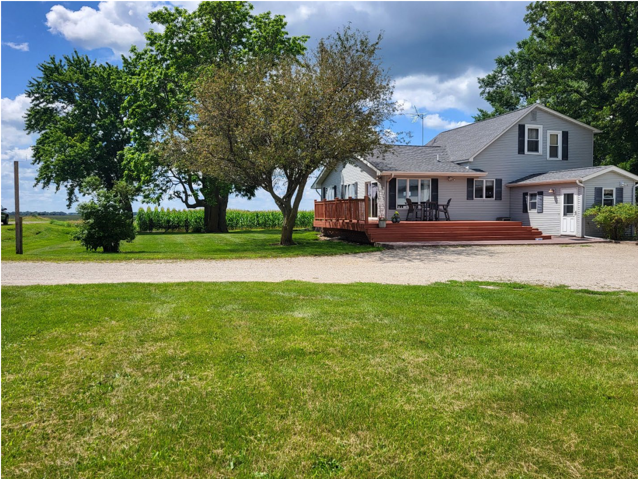
Figure 3 – looking south at house and existing deck
