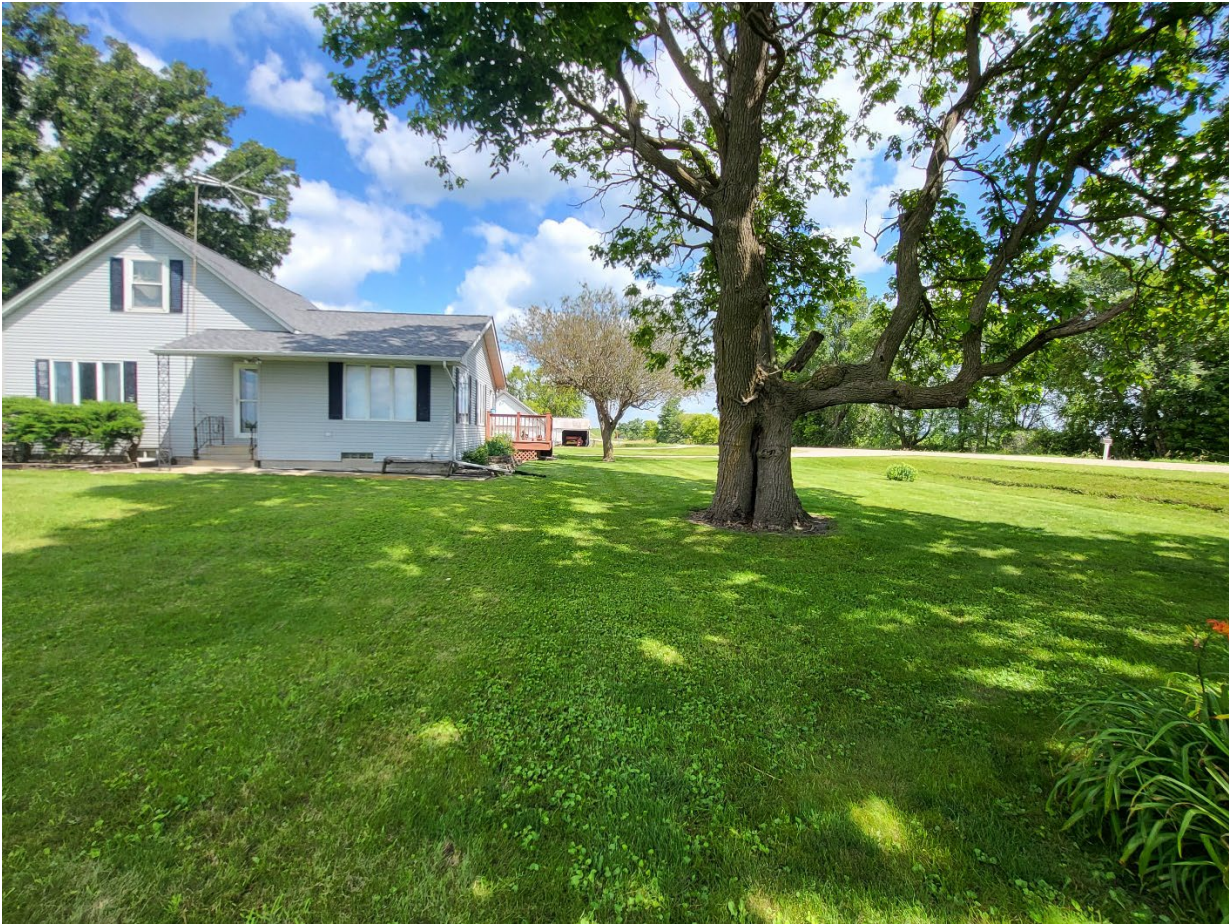
Figure 2 – looking north at house and existing deck
