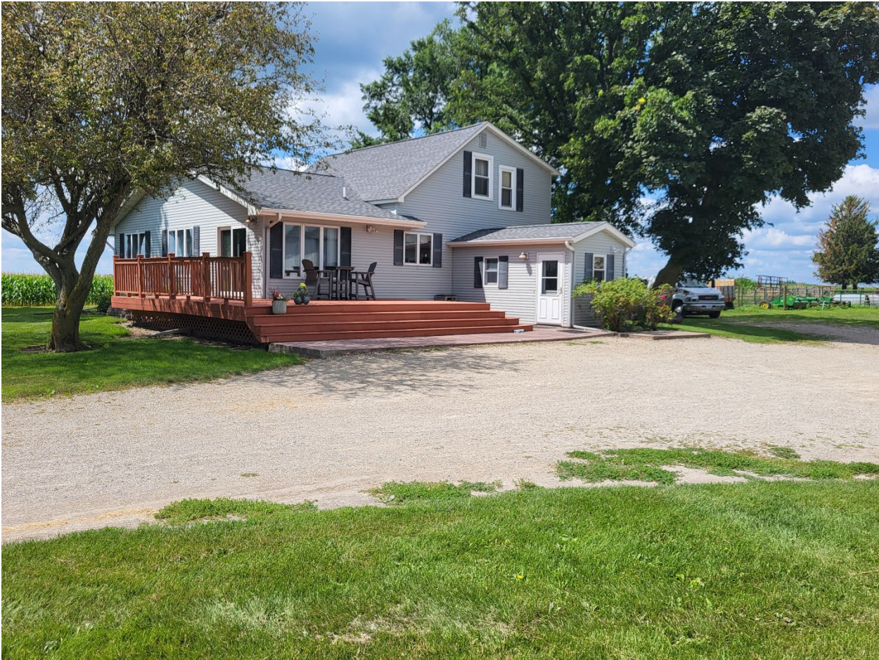
Figure 4 – location of proposed breezeway and attached garage on north side of house
