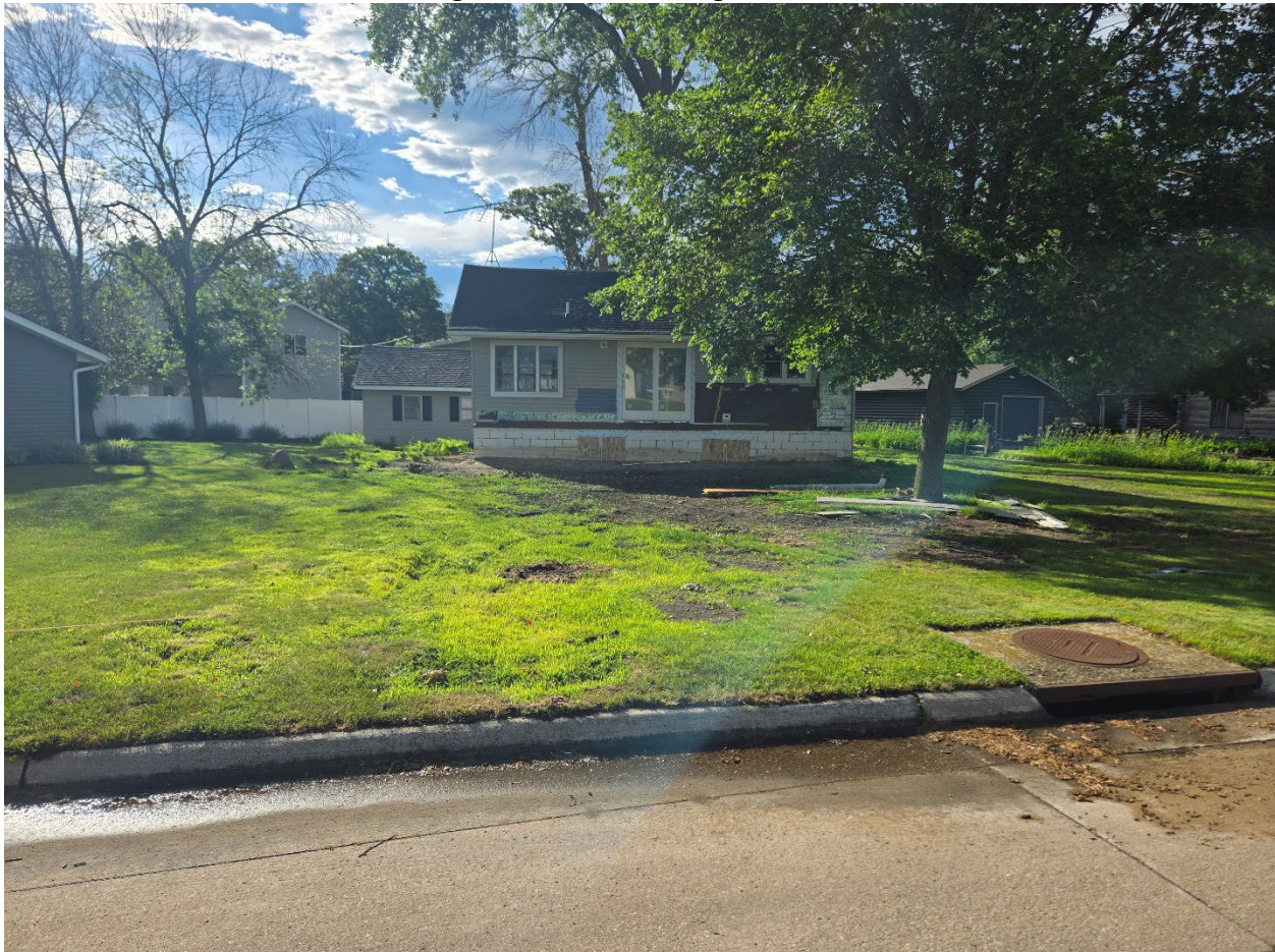
Figure 1 Looking at front of dwelling from Crane St
