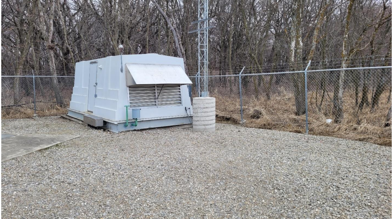
Figure 1 Looking at the site of the proposed improvements
