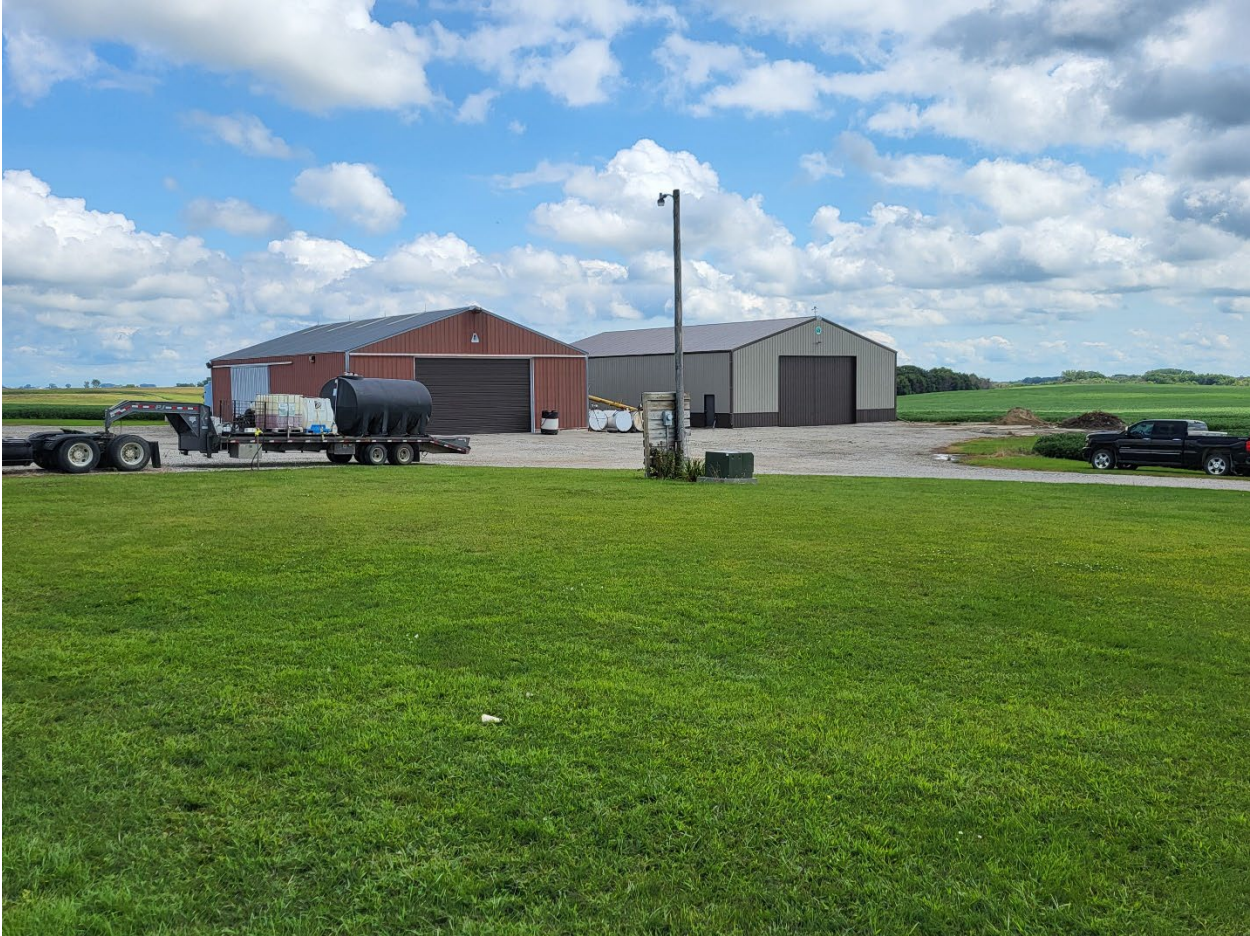
Figure 3 Looking at machine sheds
