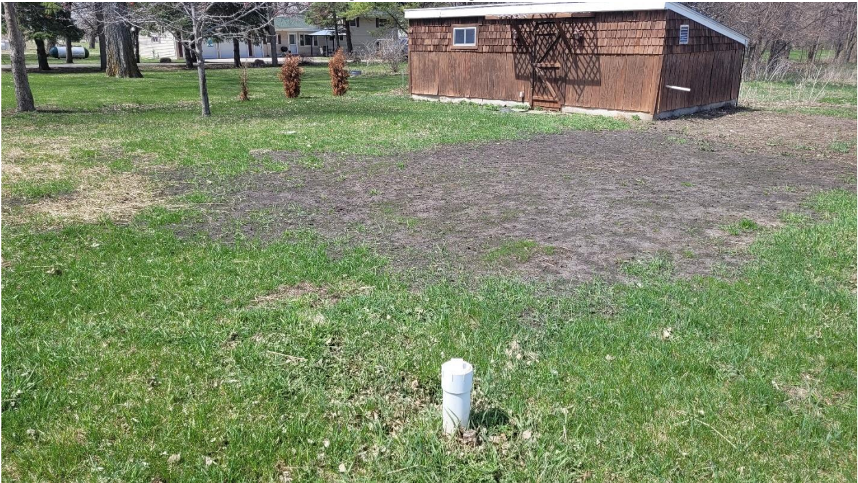
Figure 8 Looking at the existing leech field
