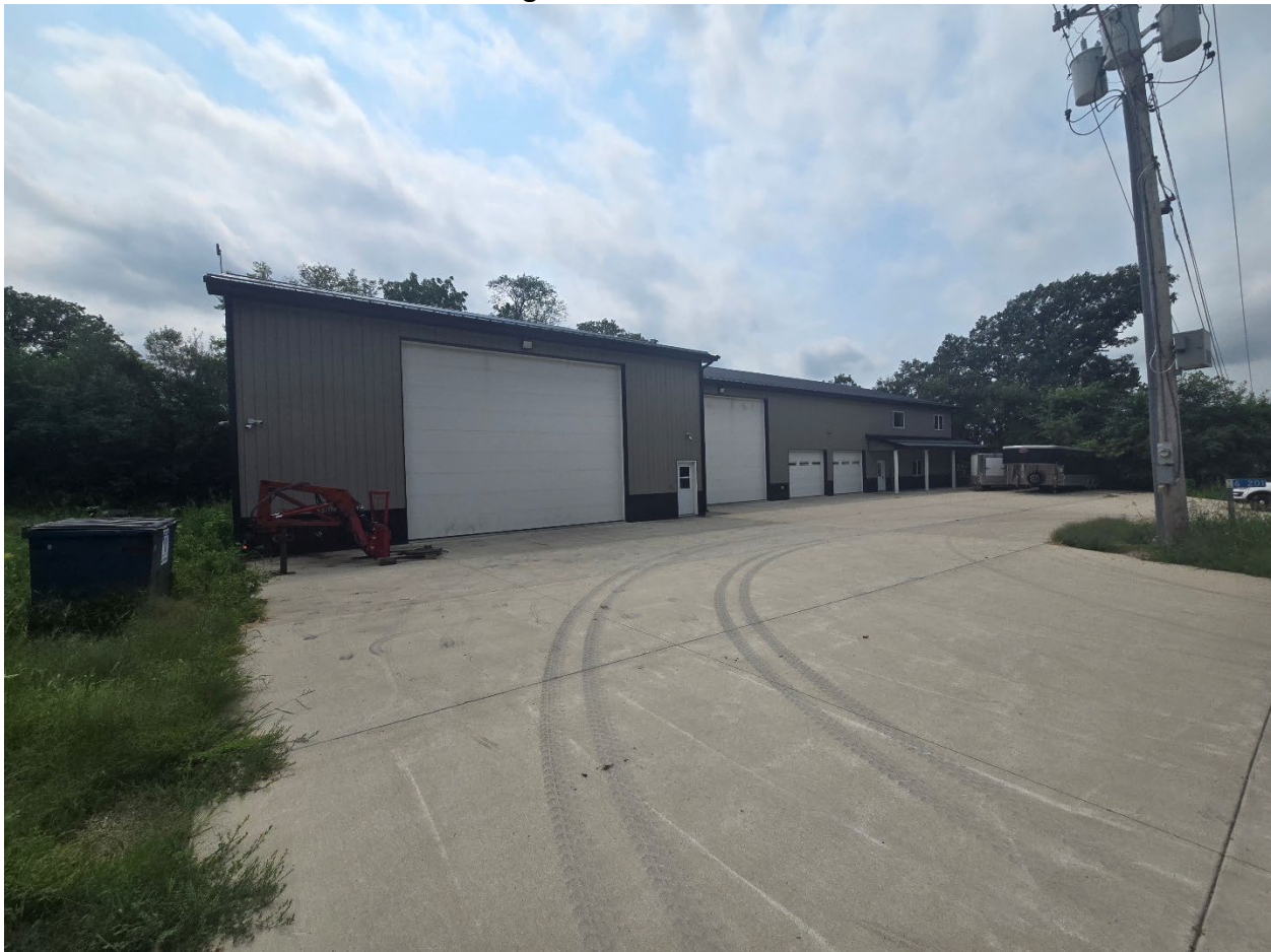
Figure 1 Existing structure from Southshore Dr
