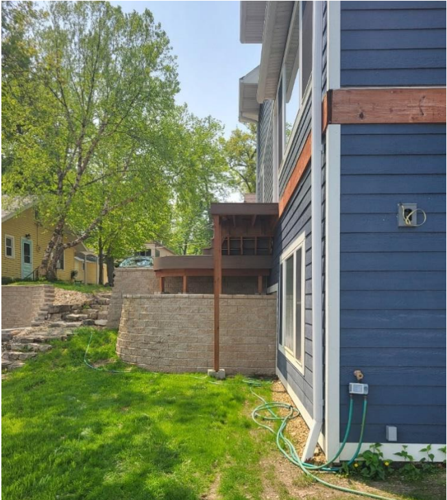
Figure 4 – looking south showing location of walkway on front of house
