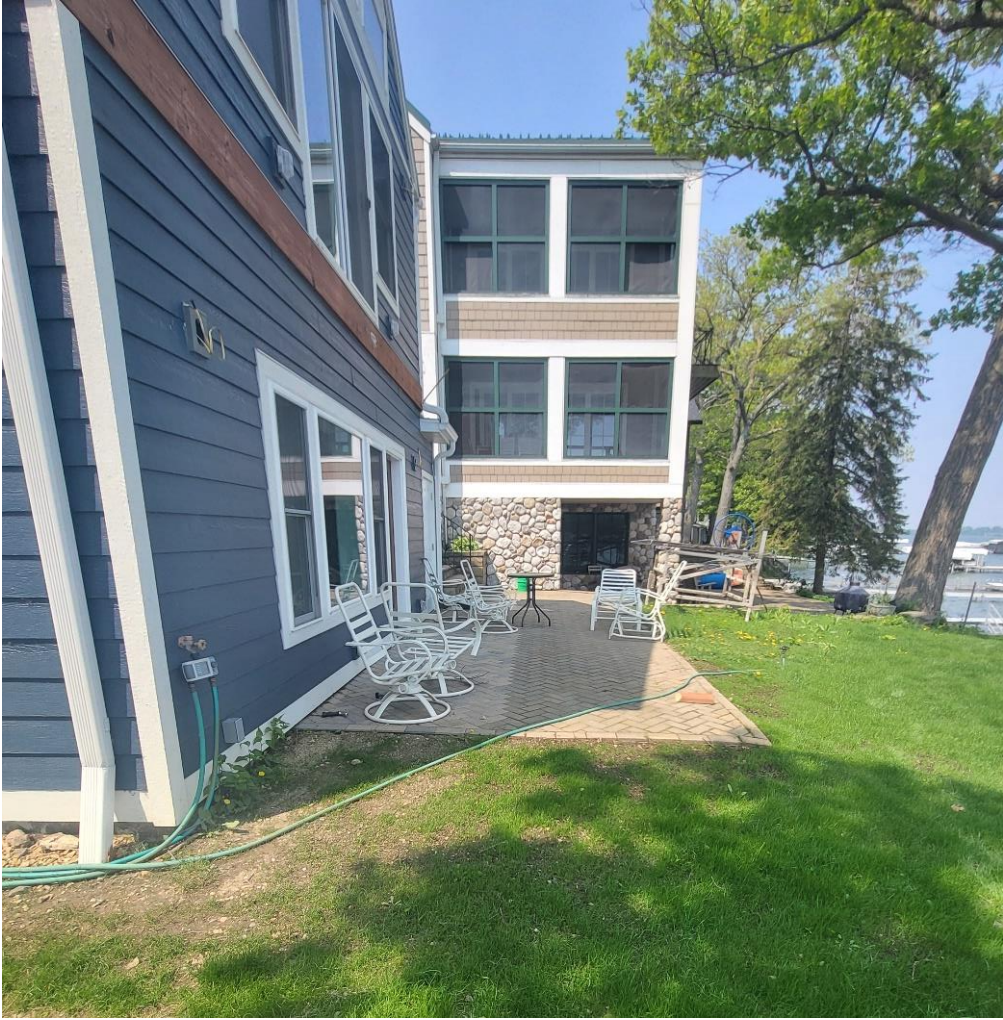
Figure 3 – looking along deck footprint in relation to neighbors house to the west
