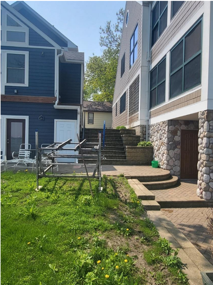
Figure 5 – looking south along the rear (west) lot line
