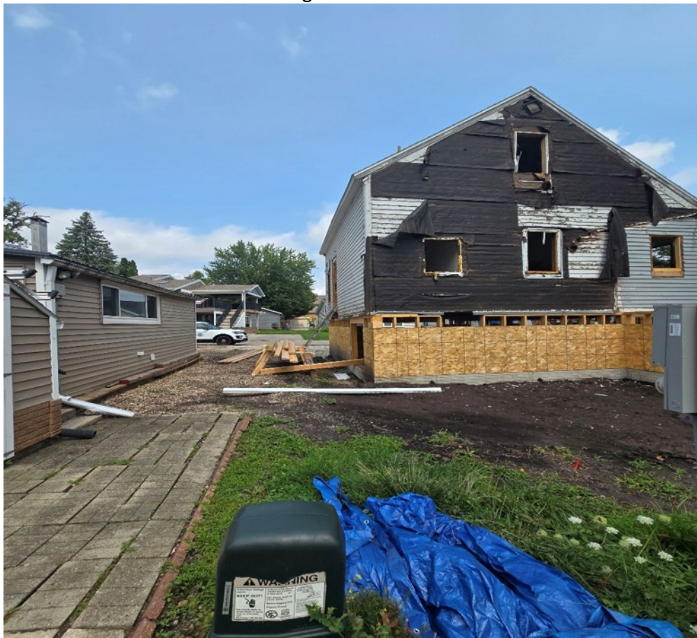
Figure 3 Looking at rear of house
