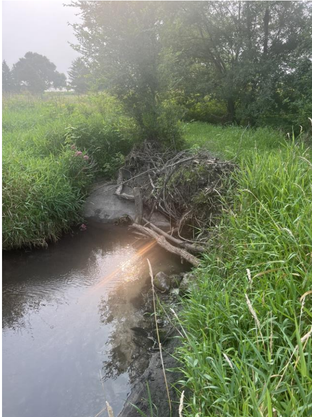
Figure 1 Upstream Side of Crossing
