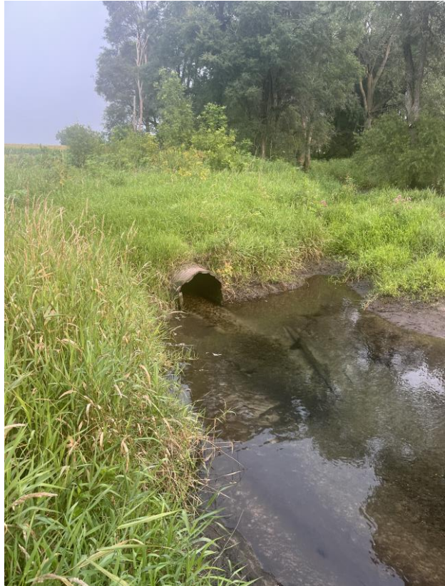
Figure 2 Downstream Side of Crossing
